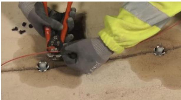
Tighten with a 12mm (1/2") ring spanner ring spanner. Twist the excess wire from the PatchGuard Connect units around the titanium feeder wire to ensure electrical continuity.
