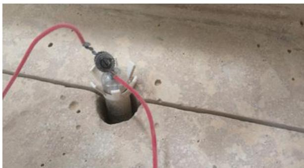
Check the connection between the PatchGuard Connect anode and the feeder wire by using a multi meter to ensure a resistivity of 0.5 ohm or less.
