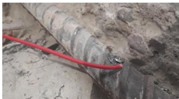
5. Remove dust and debris and then, using a spray bottle or other suitable method, wet out the holes for a **minimum of 15 minutes** ensuring that any excess water is removed prior to application of the DuoCrete PG mortar.
