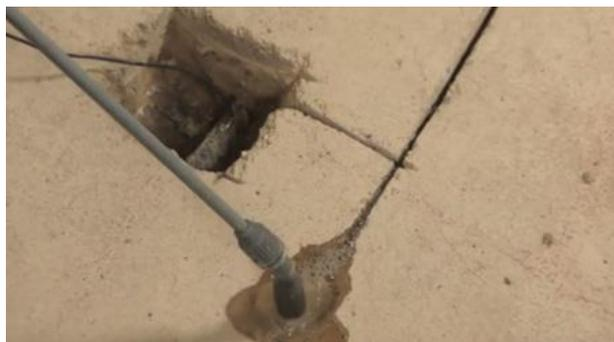
6. Strip the coating from the titanium wire using wire strippers, only in the location where the anodes are to be fixed. With the PatchGuard Connect anodes positioned in the holes electrically connect the individual units to the titanium feeder wire using the plastic screw connector.
