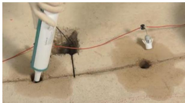
**Note: The PatchGuard Connect anodes should be installed immediately after injection of the DuoCrete PG mortar.**
