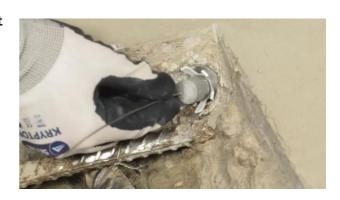
**7.** Connect the PatchGuard by wrapping the anode tying wire (minimum 2 times) around the pre-cleaned steel bar and carefully tightening using pliers.
