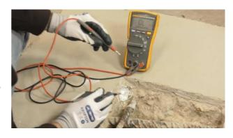
Repeat this process until a resistance of 0.5 ohm or less is achieved then secure the anode wire to the steel using 2 plastic cable ties.
