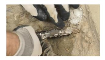
**8.** The electrical resistance between the connecting wire on the PatchGuard anode and the reinforcing steel should be confirmed to be **0.5 ohm or less.**
