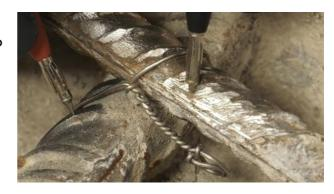
**4.** Drill 25mm (1") holes of the required depth at the edge of the patch repair (see table) making sure to avoid contact with the steel. Remove excess dust.
