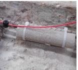
A type of DuoGuard hybrid anode used in areas of congested steel and for new construction applications.
